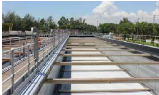
Sewage treatment plant, sedimentation tanks Siu Ho Wan, Hong Kong
