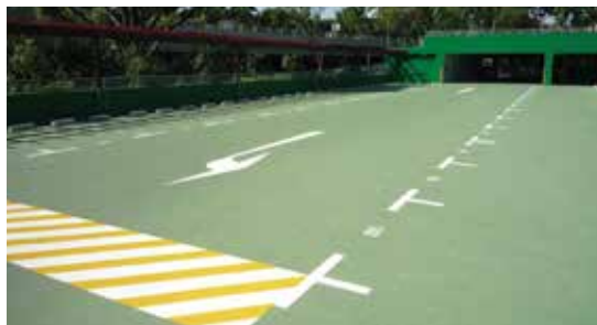
MasterSeal Traffic 2500 HD MacRitchie reservoir car park, Singapore
