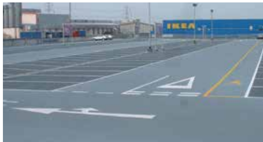
MasterSeal Traffic 2500 HD IKEA Leeds, United Kingdom
