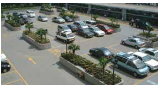
MasterSeal Traffic 2500 HD HKCLK Airport car park, Hong Kong
